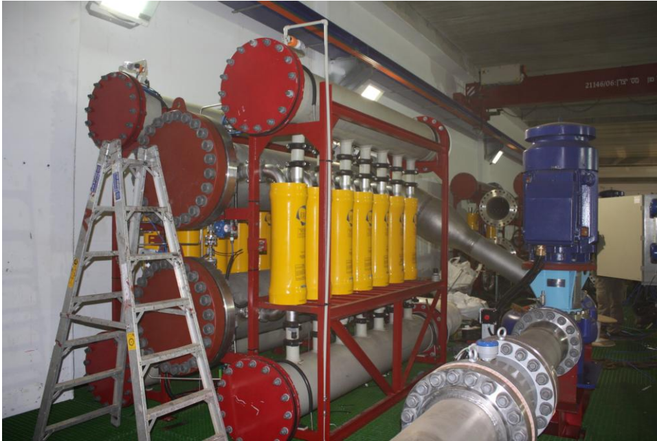
Figure 6 ERD during installation.
