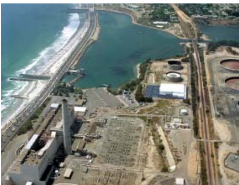
Figure 2. Carlsbad Seawater Desalination Project
