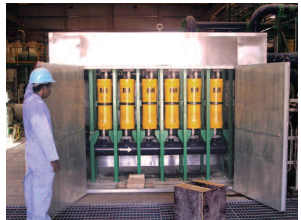
FEWA, UAE, 5,000 m 3 /day Modular Rack Assembly with Sound Enclosure
